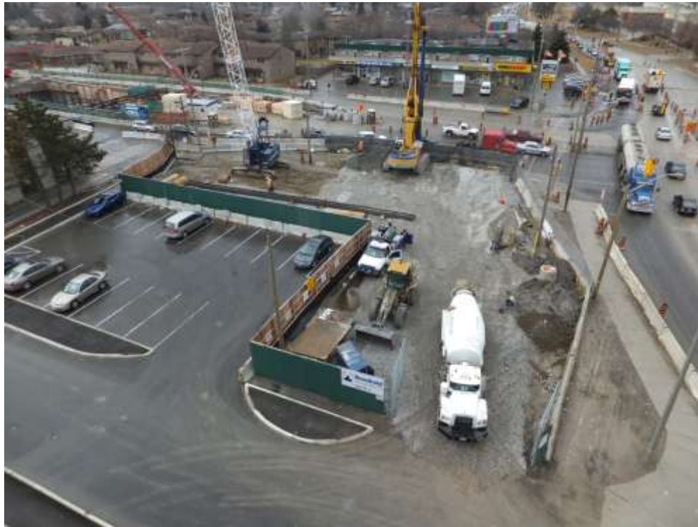
Subway construction at Keele and Finch: Just one lane each way, for multiple years.
