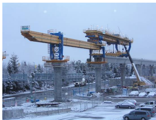
Beams can be assembled in segments on site and put into place using precast segmental construction method.
