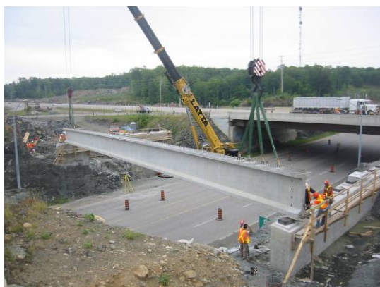
Beams can be transported to the site on a truck and then lifted into place with a crane
