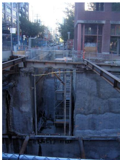
Area is excavated down to track level. To minimize impacts, soil retention systems are used.
